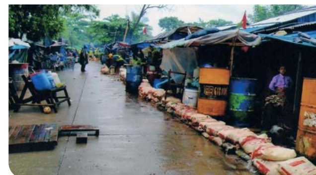
Flood protection by sandbags in North Okkalapa and Dagon Myothit (South) Townships Photo: Drainage and Sewerage Management Department
